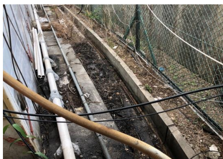
(Observed on 18 Feb 2020)
