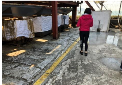
(Observed on 18 Feb 2020)
