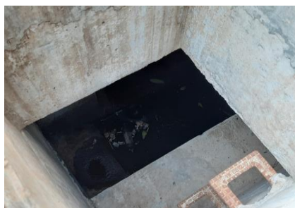
(Observed on 18 Feb 2020)
