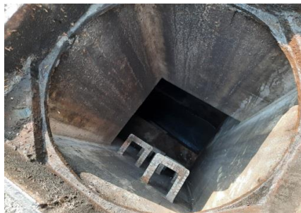
(Observed on 18 Feb 2020)
