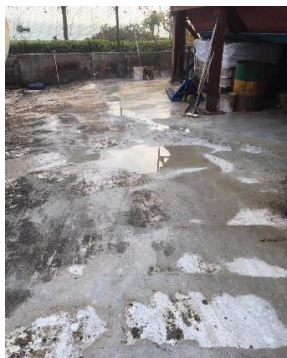
(Rectification work on 19 March 2019)
