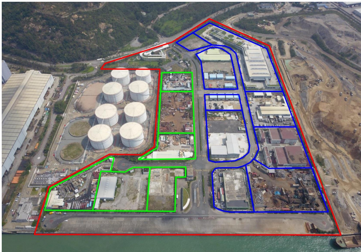
Figure 1-1 Location of EcoPark in Tuen Mun Area 38
