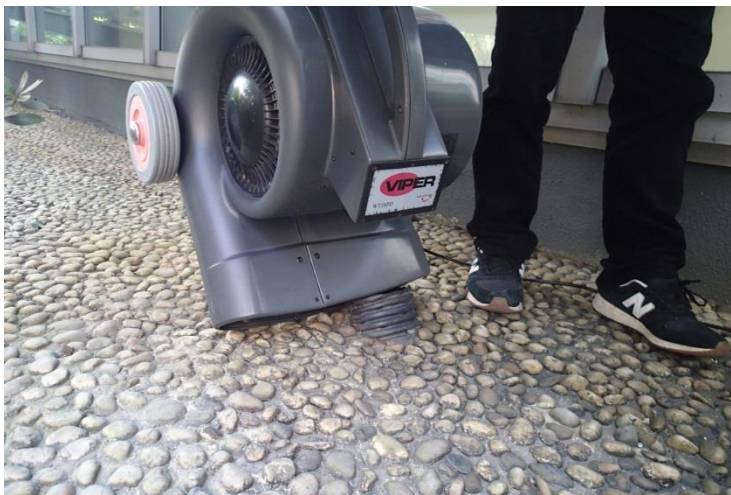
Figure 5-1 Cleaning of Underground Utilities in December 2017
