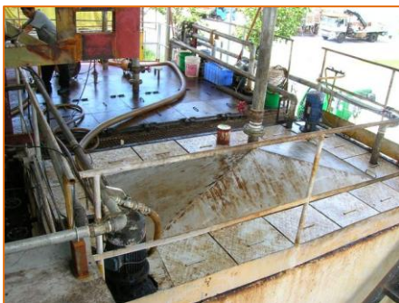
Photo 1 Covers of the Oil/Water Mixture Storage Tanks and Surplus Water with Dregs Storage Tank Remained Closed
