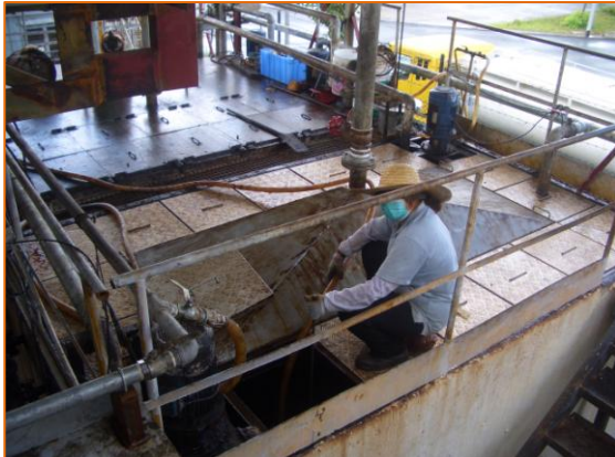
Photo 2 Cleaning or Transference of oil at the Oil/Water Mixture Storage Tanks
