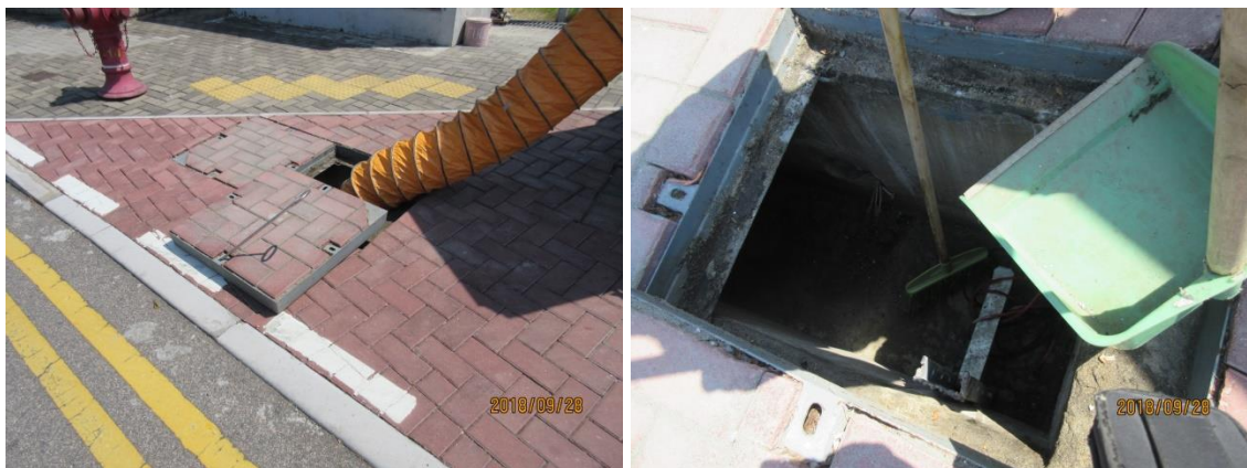
Figure 5-1 Cleaning of Underground Utilities in September 2018
