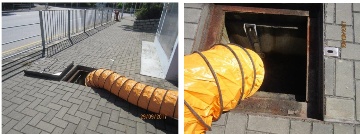
Figure 5-1 Cleaning of Underground Utilities in September 2017
