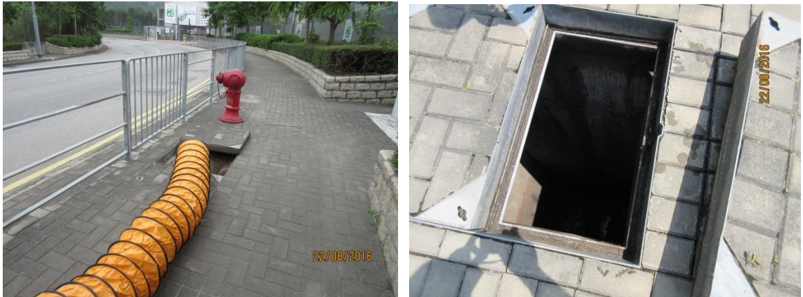
Figure 5-1 Cleaning of Underground Chambers and Utility Pipes
