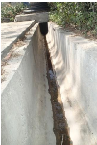
(Conditions of perimeter drains observed on 21 March 2018)
