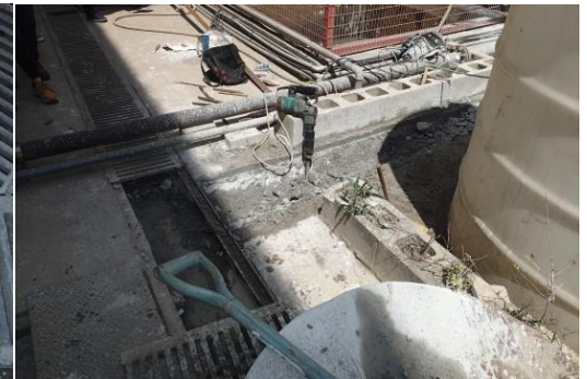
(Surface channel construction observed on 21 March 2018)
