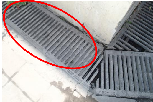
(Raised invert level observed on 21 March 2018)
