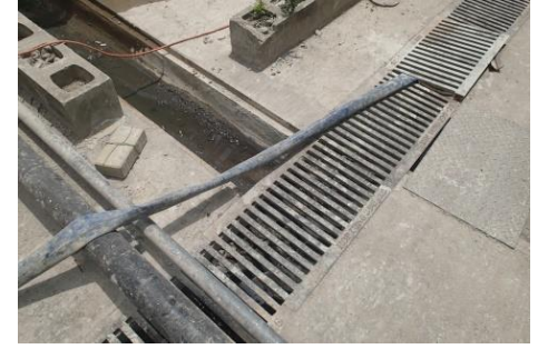
(Surface channel construction observed on 16 May 2018)
