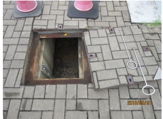
Figure 5- 1 Cleaning of Underground Chamber and Utility Pipe
