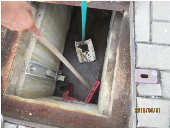
Figure 5- 1 Cleaning of Underground Chamber and Utility Pipe
