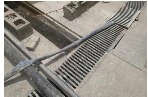
(Surface channel construction observed on 16 May 2018)
