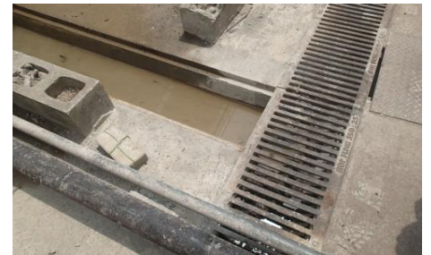
(Surface channel construction observed on 19 April 2018)
