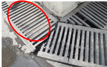
(Raised invert level observed on 19 April 2018)
