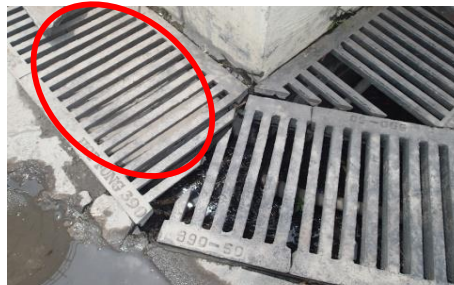
(Raised invert level observed on 19 April 2018)
