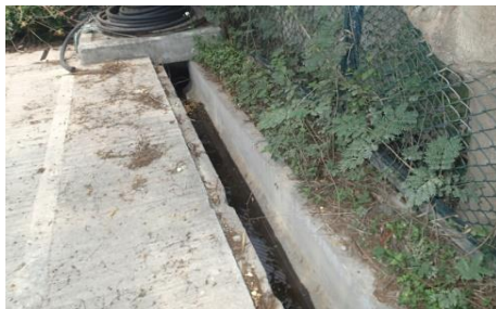
(Conditions of perimeter drains observed on 19 April 2018)
