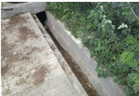
(Conditions of perimeter drains observed on 16 May 2018)
