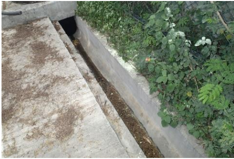
(Conditions of perimeter drains observed on 16 May 2018)
