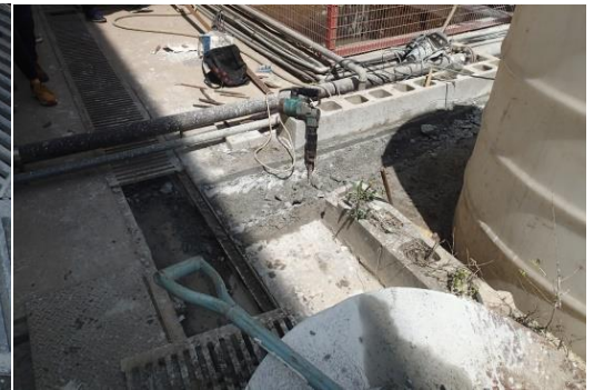
(Surface channel construction observed on 21 March 2018)
