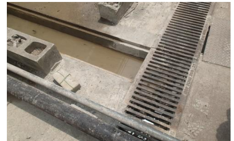
(Surface channel construction observed on 19 April 2018)
