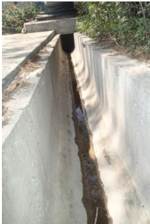
(Conditions of perimeter drains observed on 21 March 2018)
