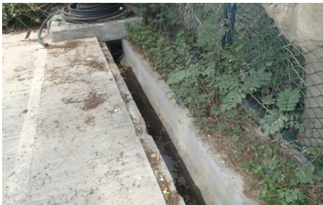
(Conditions of perimeter drains observed on 19 April 2018)
