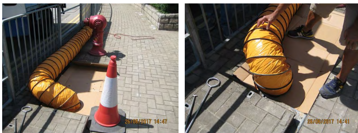
Figure 5-1 Cleaning of Underground Chamber and Utility Pipe
